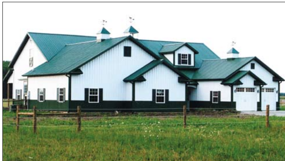
Figure 24. Although any exterior finish may be used, steel siding and roofing are popular due to economy and maintenance-free durability.
