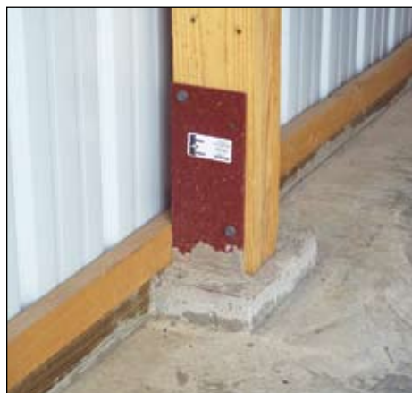
Figure 15. Cast-in-place concrete piers may be used for post-frame buildings.
