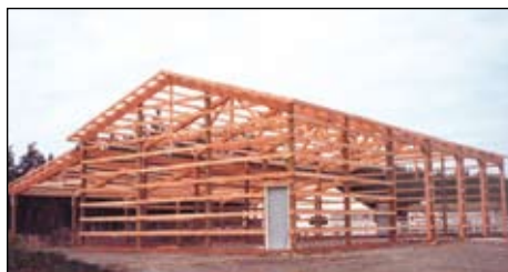
Figure 10. A typical post-frame building frame.
